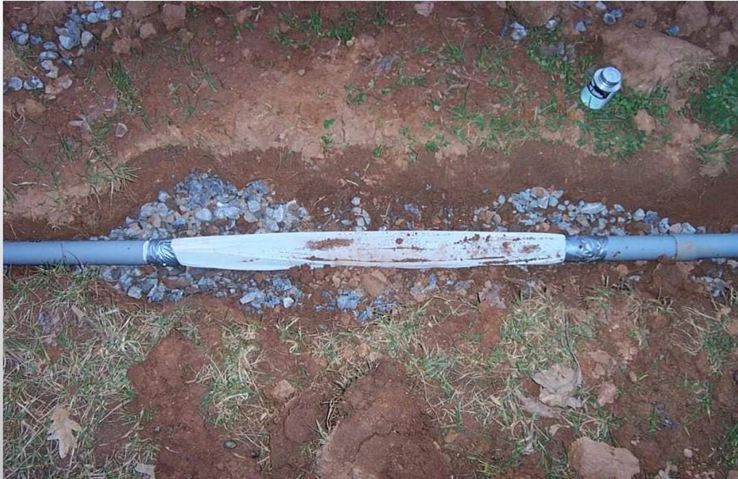
*At the lowest point of the conduit run, I created a French drain. Water will get into the conduit, even from condensation. It needs a way out.*
