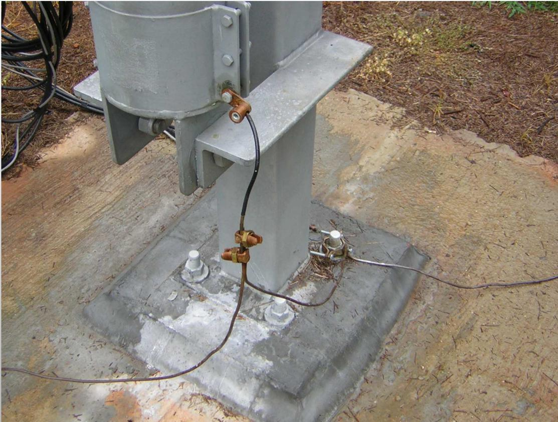
*NEVER let copper wire and your galvanized tower touch. Don't even let rain drip from copper wire to the tower. It will corrode your tower. Use brass or stainless steel transition clamps to bond to the tower.*
