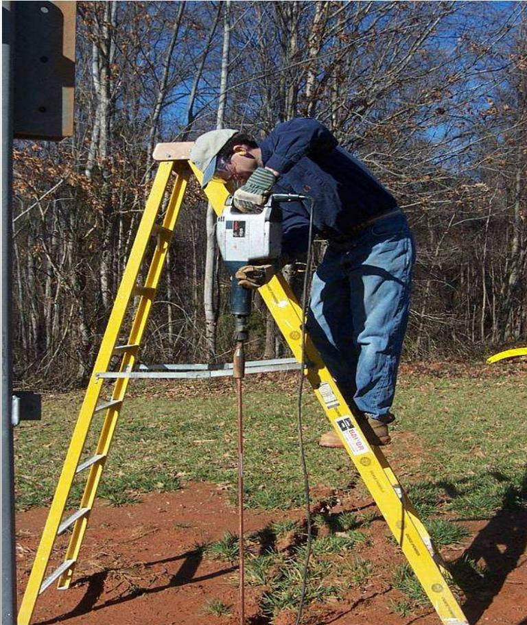
*Rent a rotor-hammer with a ground rod bit. It makes ground rod installation easy even in hard Carolina clay.*
