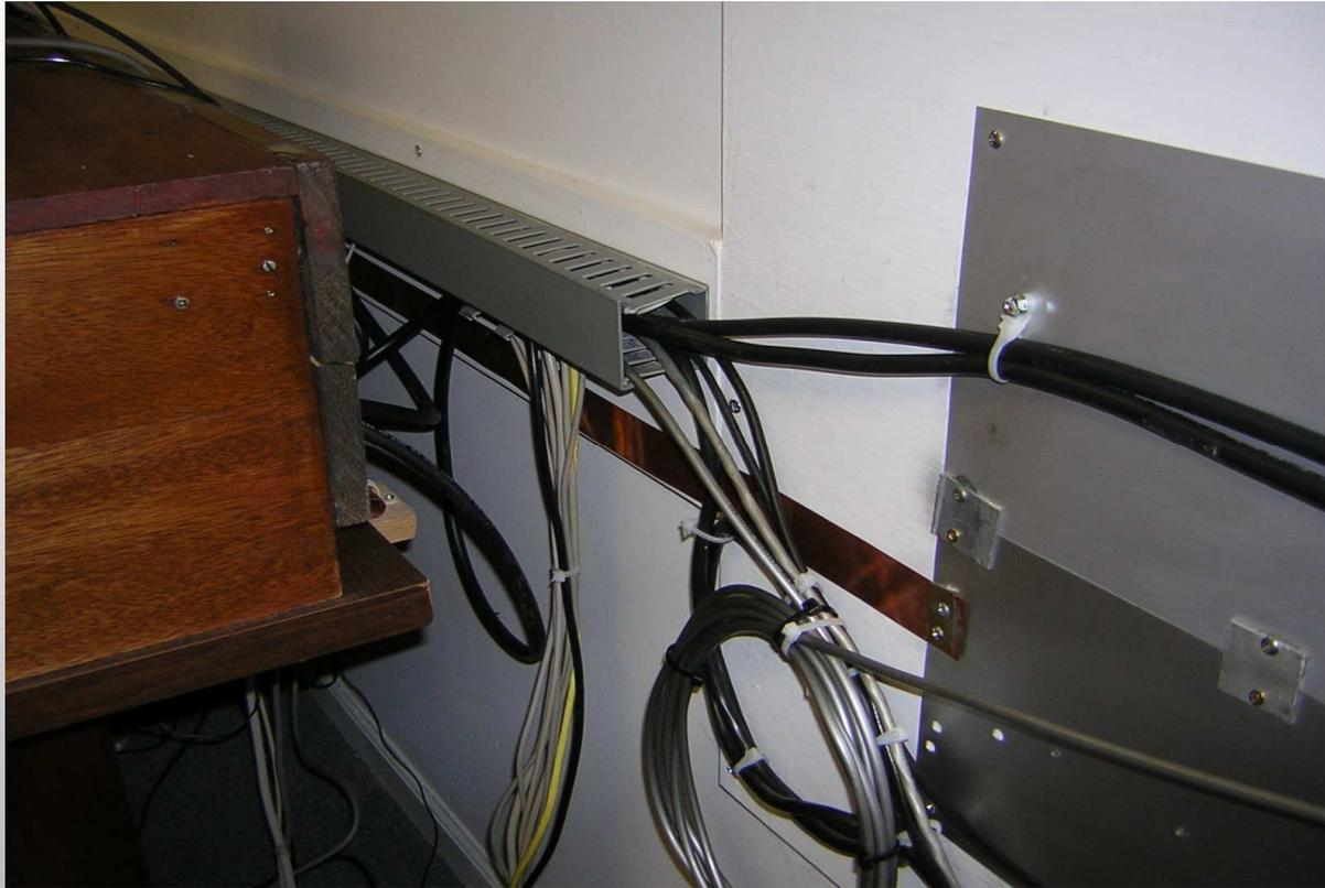
*1.5" copper strap run behind radio desk for bonding equipment to ground. Then the strap is bonded to the kick plate. Copper pipe works well too.*
