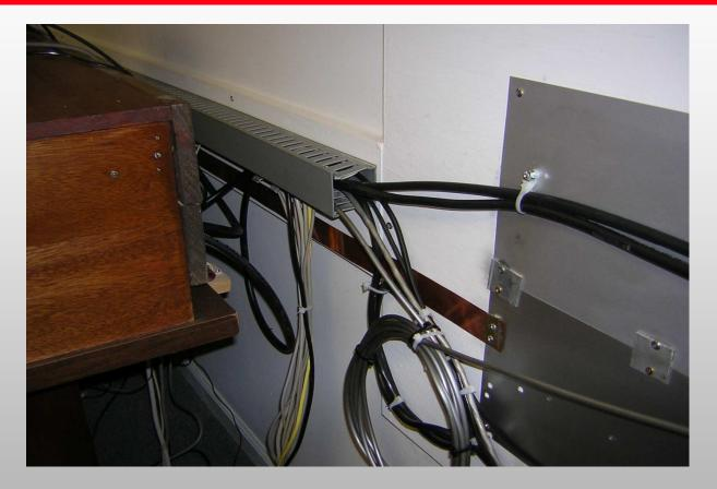
1.5" copper strap run behind radio desk for bonding equipment to ground. Then the stap is bonded to the kick plate. Copper pipe works well too.
