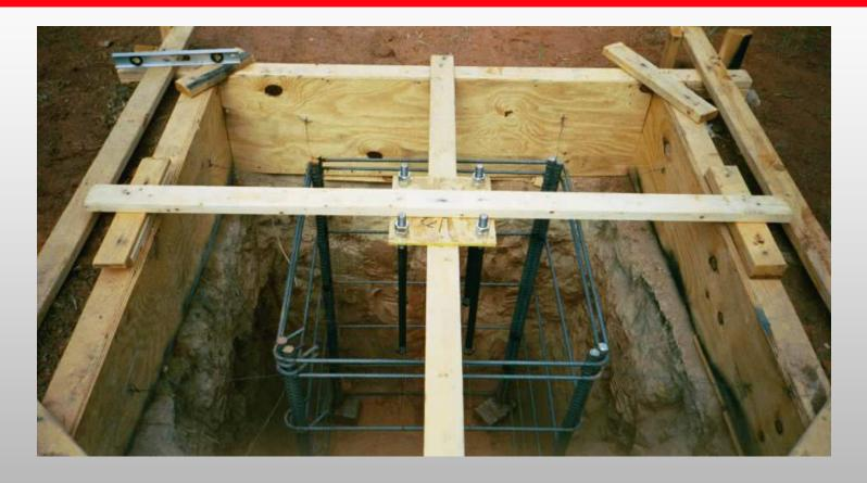
Make sure the re-bar cage isn't resting on the ground into the dirt. Set it off the ground on bricks or concrete blocks. The concrete must completely cover the re-bar or it will rust away..
