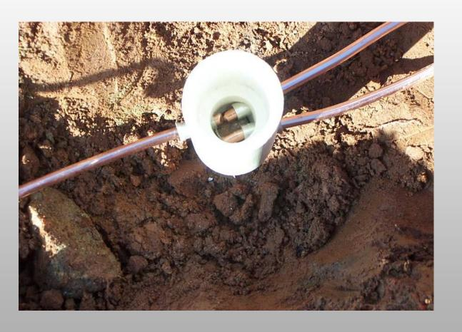
Use exothermic connections to create a permanent bond between the ground wire and the rod. I used Cadweld "One-Shot's"
