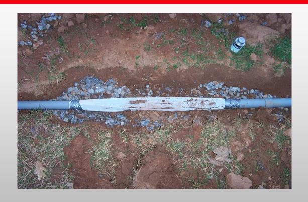
At the lowest point of the conduit run, I created a French drain. Water will get into the conduit, even from condensation. It needs a way out.
