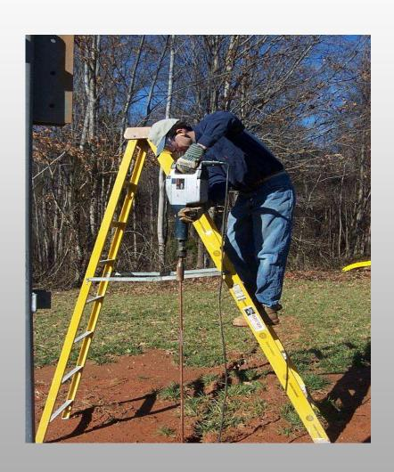
Rent a rotor-hammer with a ground rod bit. It makes ground rod installation easy even in hard Carolina clay.
