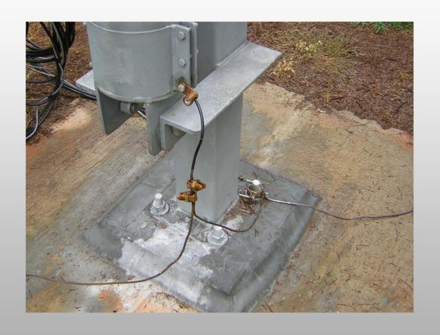
NEVER let copper wire and your galvanized tower touch. Don't even let rain drip from copper wire to the tower. It will corrode your tower. Use brass or stainless steel transition clamps to bond to the tower.
