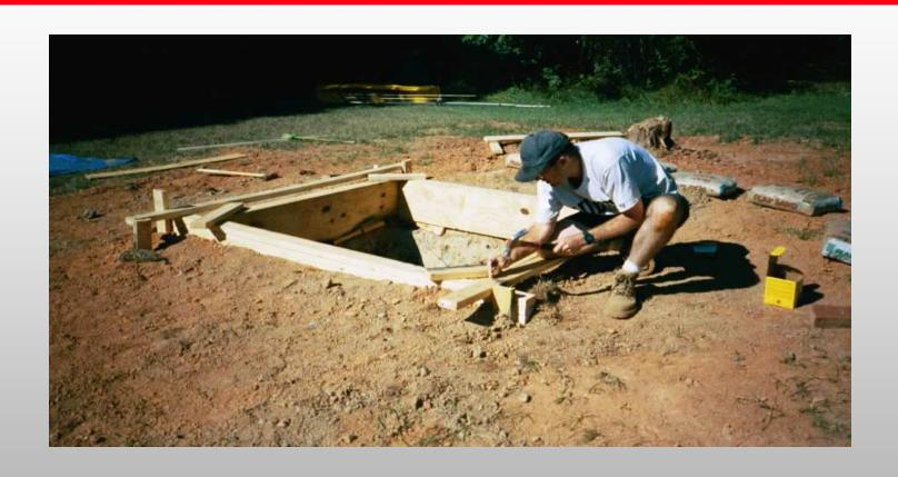
Anchor the form with stakes so the concrete doesn't push it apart.
