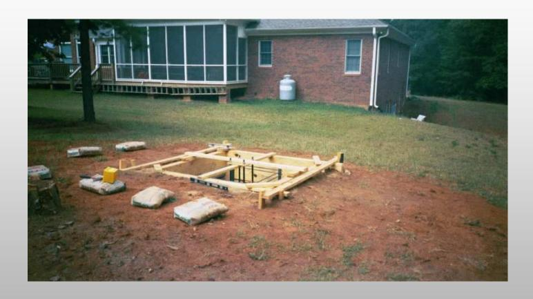
Make sure the anchor bolts are plumb and secure. The concrete and vibrator may push them out of position if they aren't tied securely.
